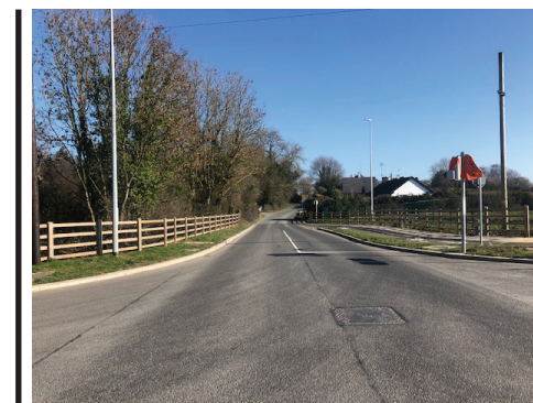
New road junction
